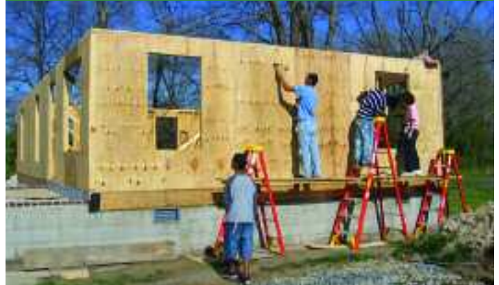
Patricia Berdan and her sons work on a Habitat home.
